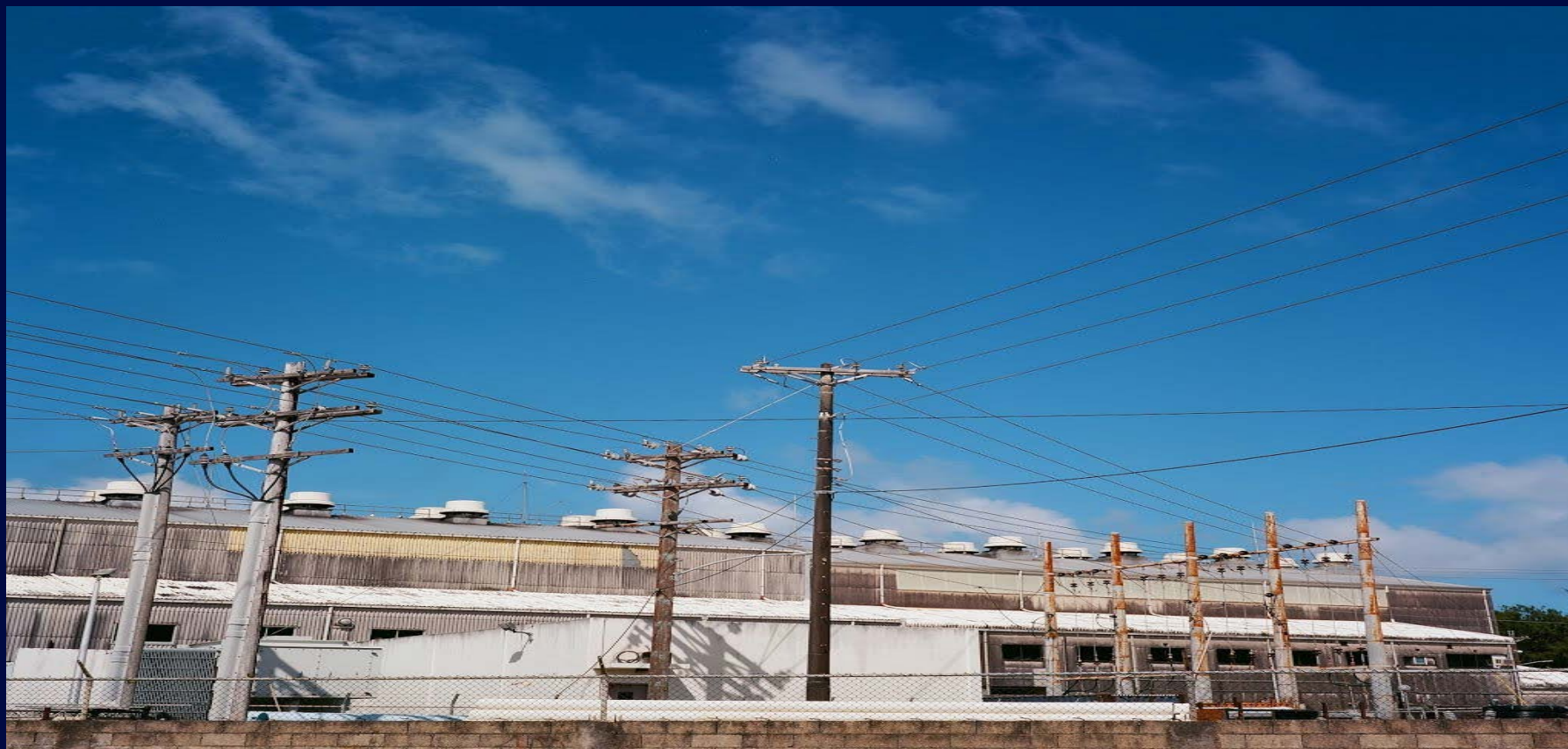
CNMI POWER PLANT
